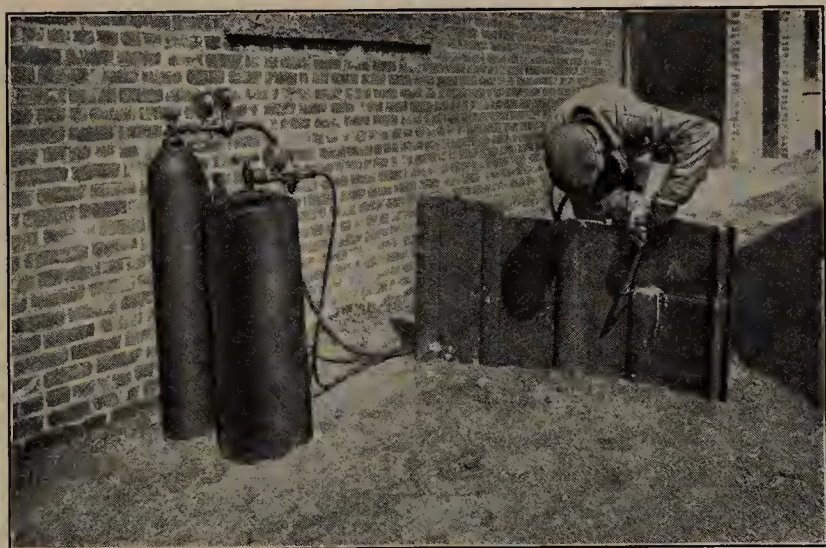
FIG. 115. Cutting an iron plate by means of the oxyacetylene blowpipe
